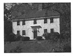
massive central chimney and a typical Georgian style door surround. The 5 bay façade, central doorway flanked by pilasters supporting an entablature, 5 light transom above the door, hipped roof, and center chimney of the house illustrate the Georgian style popular during that period of time.
