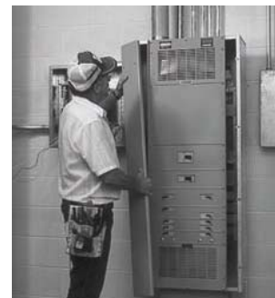
The Three-Piece Trim for Larger Power Distribution Panelboards Provides for Easy Handling and Installation
