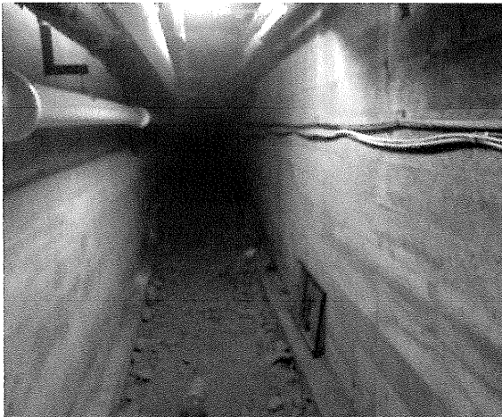
Photo #9: Windows in tunnel
