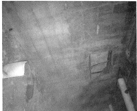
Photo #10: Windows in tunnel
