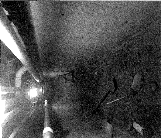
TSI debris on floor in tunnel
