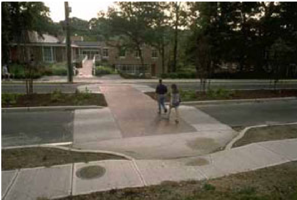
Figure 2: Raised pedestrian crosswalks can control vehicle speeds on local streets at pedestrian crossings
