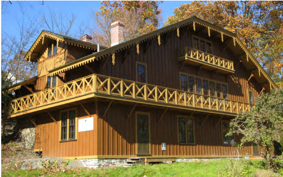
Restored façade of the Swiss with corrected paint colors
