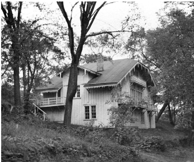
Historic photo of the Swiss Factory Lodge
