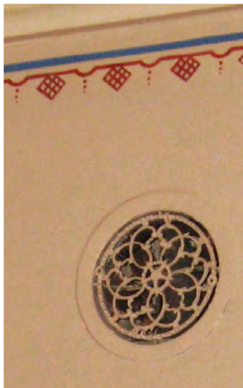
Decorative wall grille of original passive ventilators put back into use
