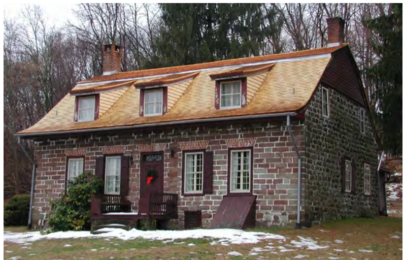
Completed roof: View from the northeast
