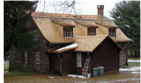
Completed roof: View from the northwest
