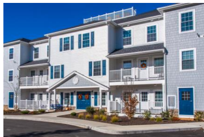
Stonington’s Spruce Manor (source: zlotnickconstruction.com)
