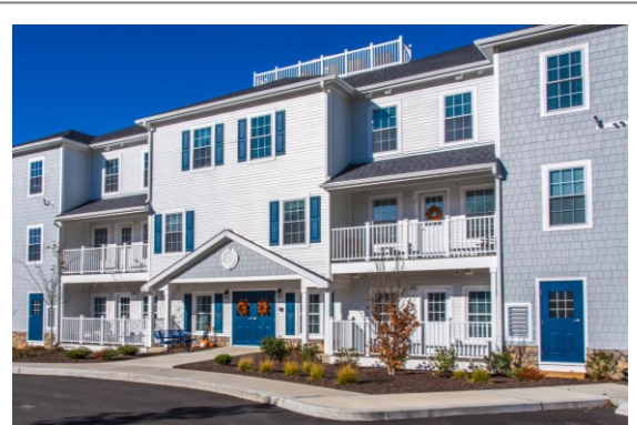
Stonington’s Spruce Manor (source: zlotnickconstruction.com)
